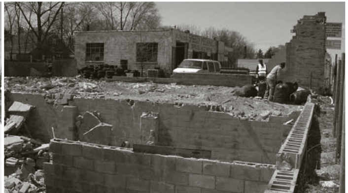
City demolition underway.
